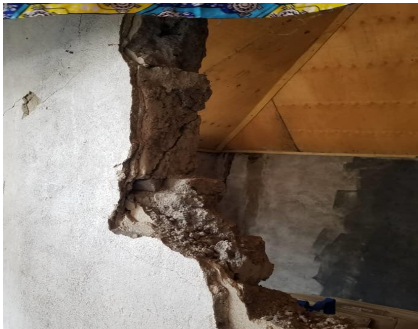
Internal walls on the first floor of the storied unit have been badly damaged
